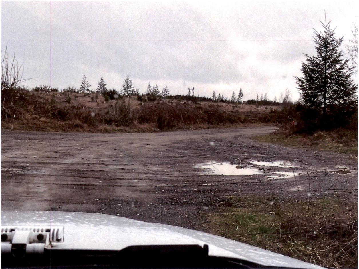
End of Maintained Section at Milepost 1.48. Note turnaround area
