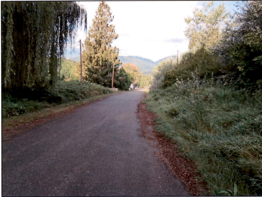
WESTERLY VIEW OF MUNCIE AVENUE, SUBJECT SITE TO RIGHT
