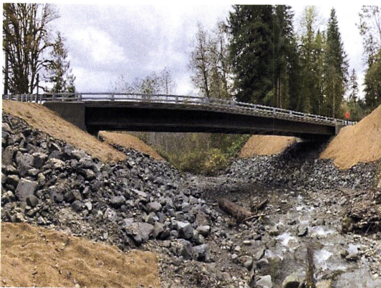
New bridge at Tower Creek (November 2022)
