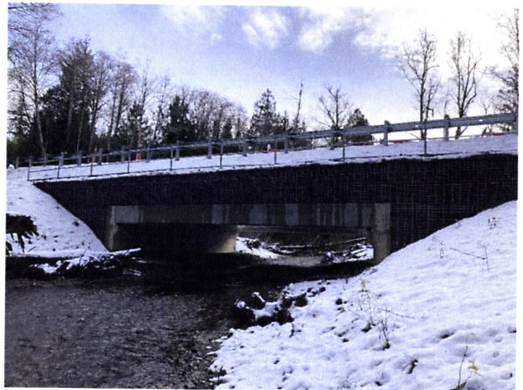
New bridge at Thorndyke Creek (February 2023)
