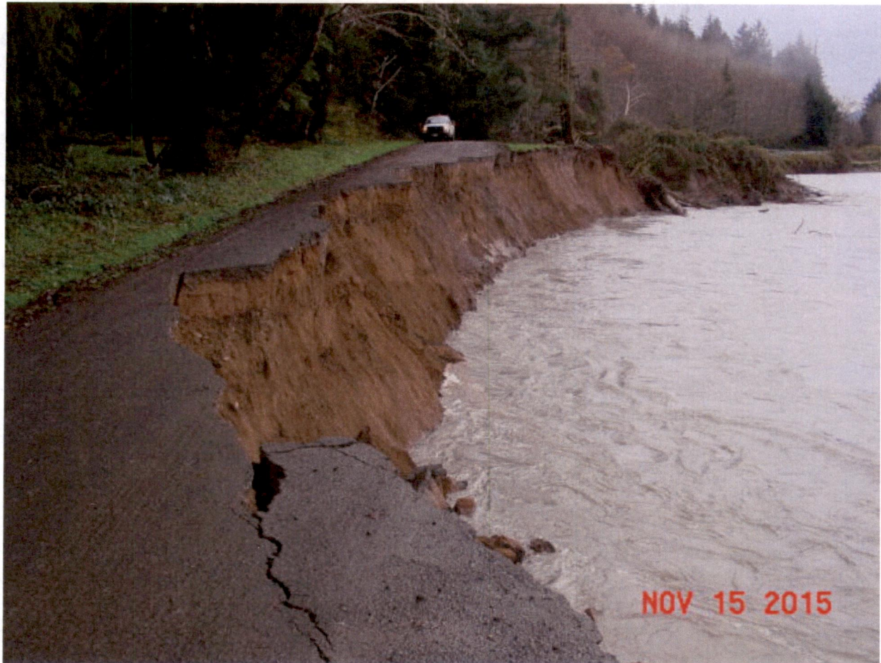
Oil City Road (2015) – Still Waiting for $500,000 from FEMA for the repair completed in 2015
