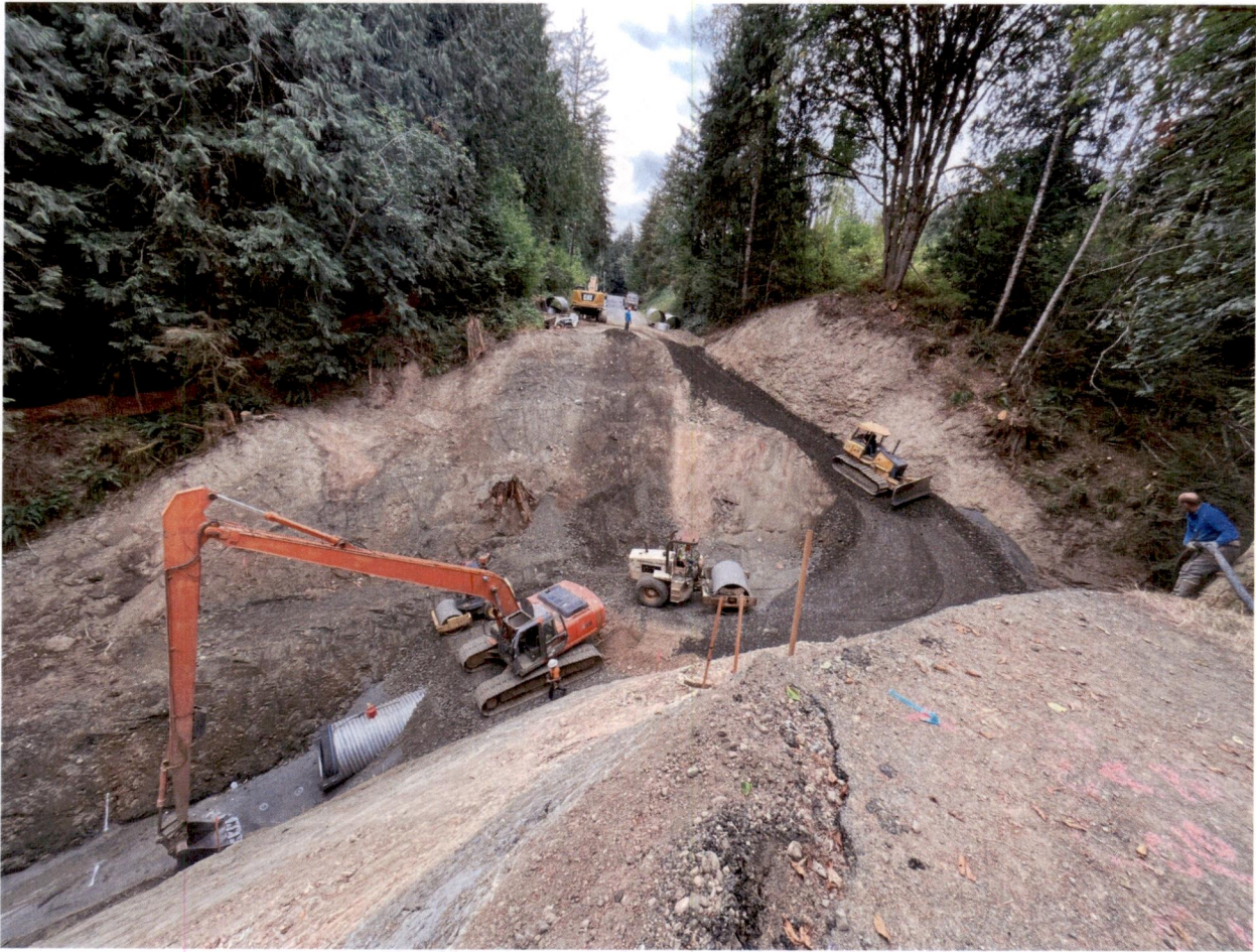
Snow Creek Culvert (2023) – FEMA Hazard Mitigation Program Success!
