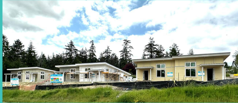
Habitat for Humanity Landes Street Project
