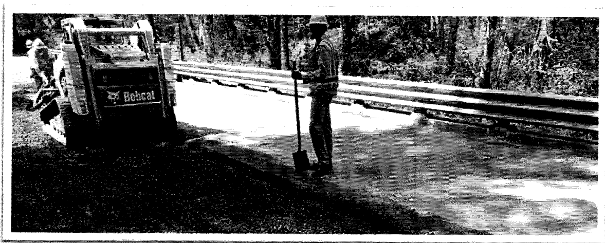
Photo - Clark County Public Works ( Milling )
