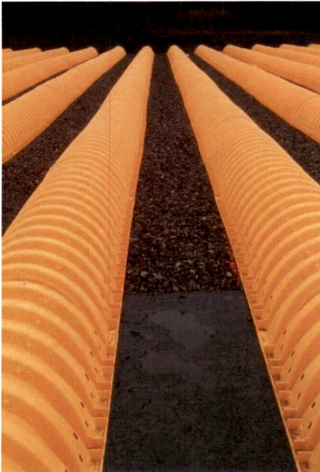
Figure 3. Construction of the Lacey/Olympia Woodland Creek Reclaimed Water Groundwater Recharge Facility (a shared water-rights mitigation project)
