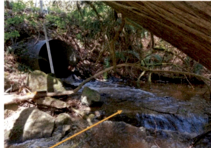
Log weirs that provided fish passage through old culvert for 40+ years
