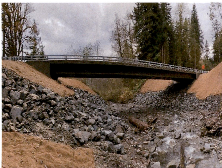
New bridge at Tower Creek (November 2022)
