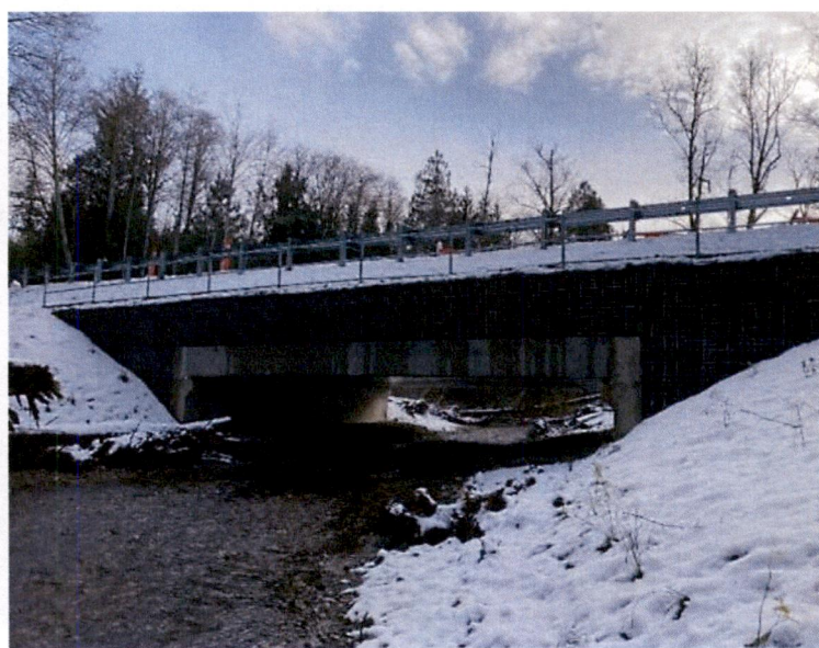
New bridge at Thorndyke Creek (February 2023)
