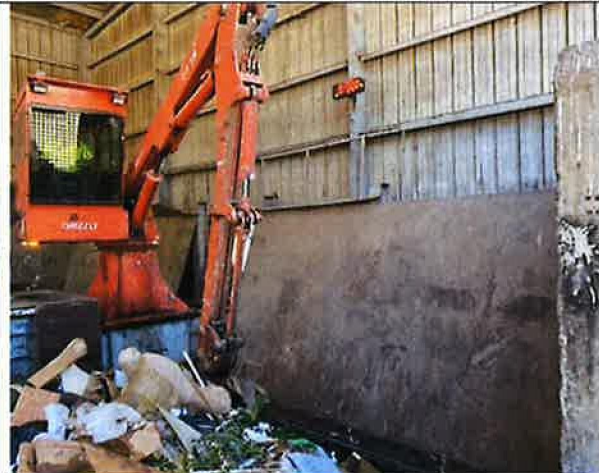
Knuckle Boom Crane (Grizzly) in Transfer Building
