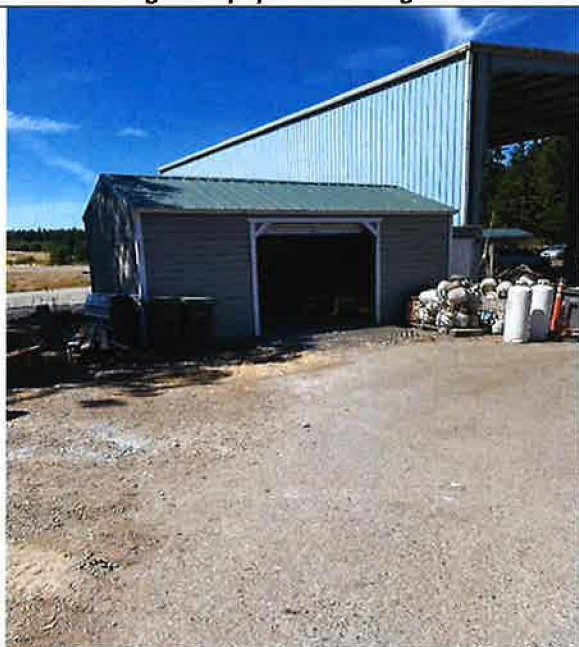
Wooden Shed adjacent to Transfer Building
