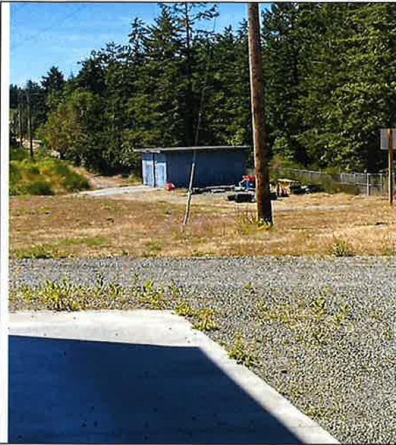
Wooden Shed West End of Site
